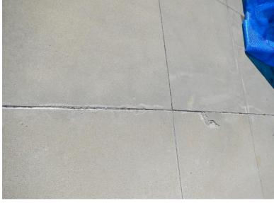
right where a significant amount of ground erosion is occurring and undermining the pool deck and adjacent light pole. The area should be repaired with filter fabric and rip rap to prevent further erosion from damaging these components.
