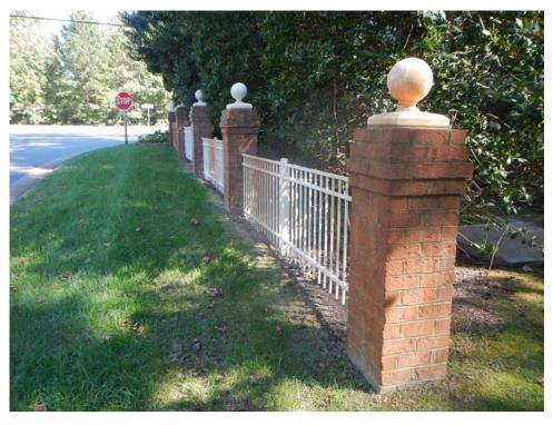
long term differential settlement of the piers and corrosion of the aluminum that weakens fasteners between members and between the fence sections and the piers.
