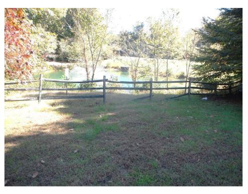
The wood split rail fencing around the club area pond is in fair to poor and failed condition. Much of the split rail fencing along the rear perimeter where the pond is fed by several inlets is missing, damaged, or fallen over. It appears as though the split rail fence was intended originally to circle the entire perimeter of the sides and rear portion of the pond and the inlets to prevent entry.
