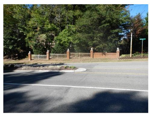
The total surface area of all the walls is approximately 2,100 s.f. Walls appear to be in serviceable condition, and they should have a very long service life. Masonry restoration and repointing will be required from time to time.
