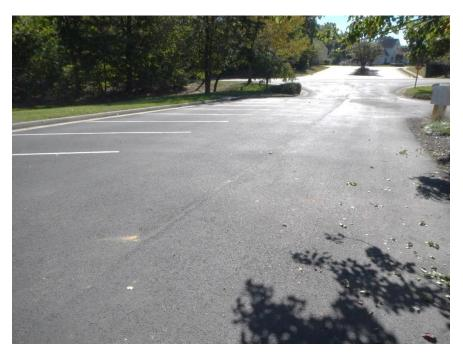
be sealed and that the entire surface be seal-coated with an asphalt sealer to protect it against harmful petroleum products from parked cars and to prolong its service life every five years or so.
